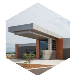
2018: Continued growth and expansion sparks the opening of the new Robert J. Warren Customer Experience Center, a 64,000 sq foot facility with multiple laboratories ideal for customer demonstrations and presentations.
